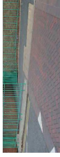
Speed humps are constructed with red brindle clay pavers within Town Centre
